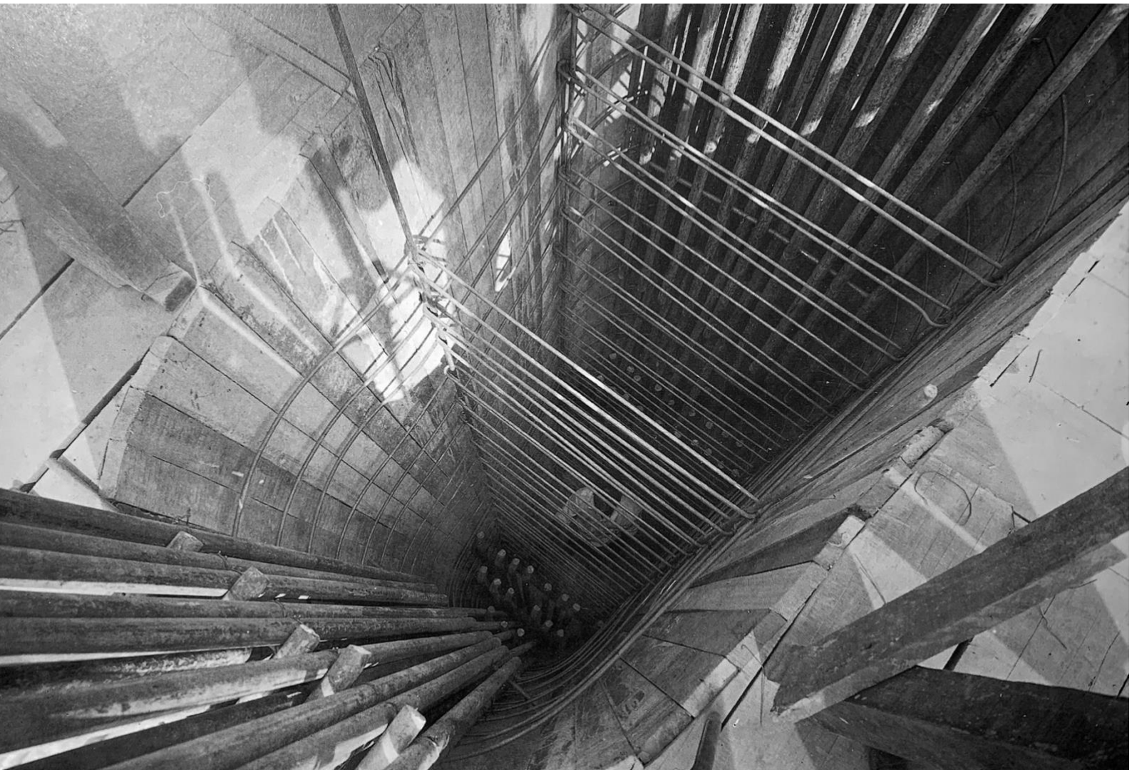
Sabena Towers in Kinshasa, Congo. Arch. Claude Laurens. 1952-54. One of the pilotis under construction
